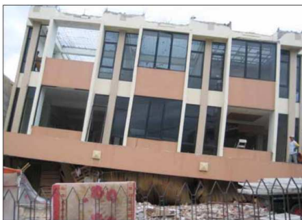
Fig. 1 Example of collapsed buildings; (a) A collapsed 3-story government building; (b) First story failure of a 3-story shop-house [1]
