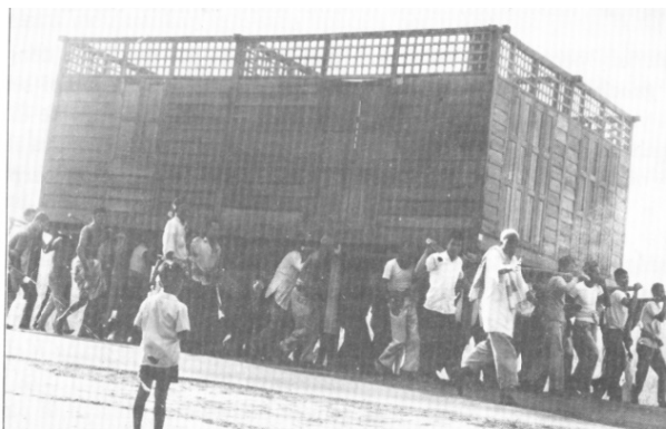
Figure 3. Traditional Malay house was move from its old site to the new site, Source: Abdul Halim Nasir 1985
