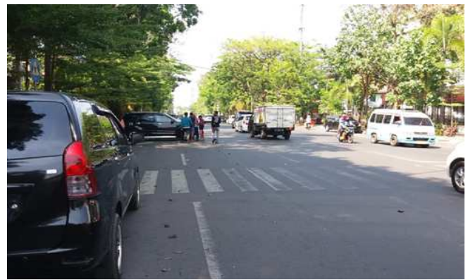
Fig. 2 The condition of the roads before the intervention
