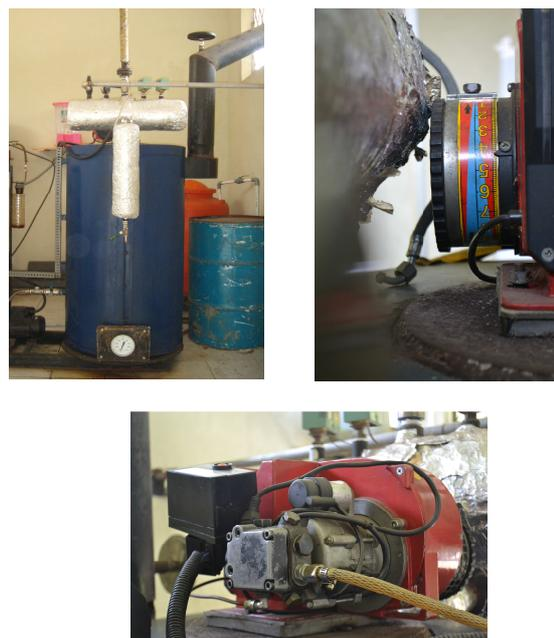
Fig. 1a. Fire Tube Boiler (1b) Burner, (1c). Fan Damper Scale
