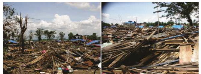
Fig. 11 Total damage due to tornado
