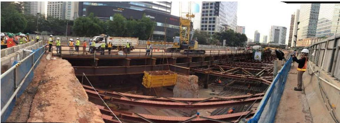
Fig. 11 Top down construction method to reduce traffic disturbance
