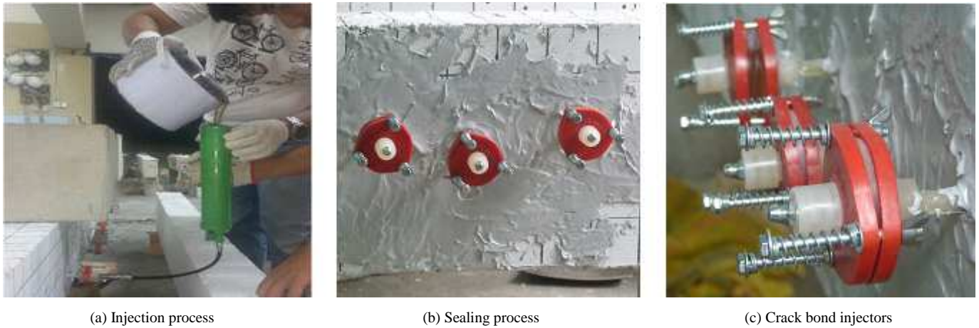
Fig. 2 The process of sealant injection method
