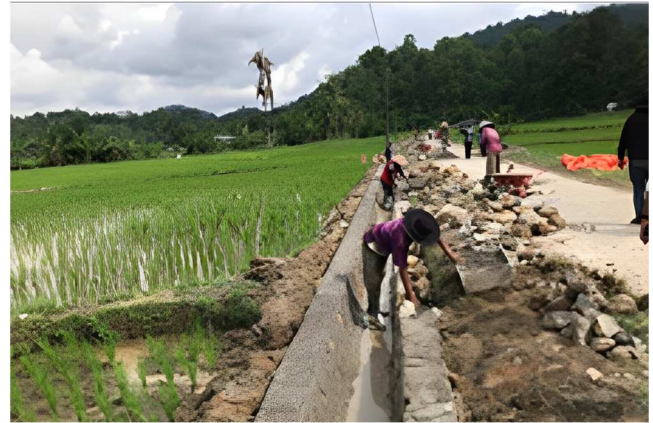
Fig. 3 Rehabilitation of tertiary channel by farmers of the P3-TGAI project
