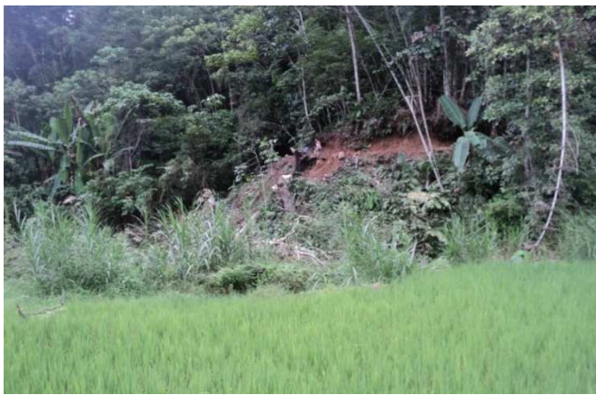
Fig. 5 Head race, forebay, and spillway constructed at the waist of the hill
