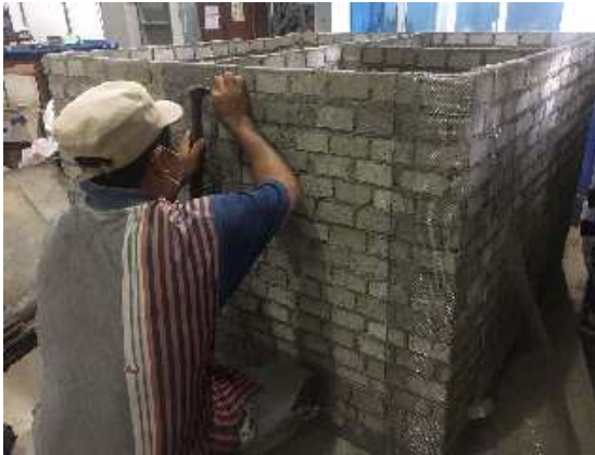
Fig. 8 Wire Mesh Installation Process
