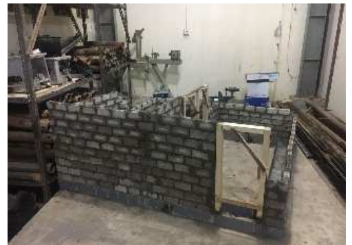
Fig. 7 Hollow Brick Wall Construction Process High 50 cm
