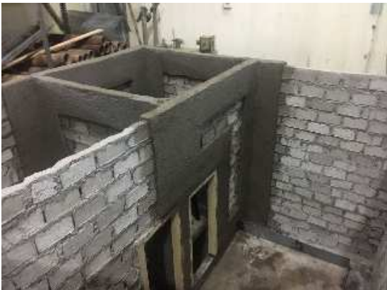
Fig. 9 Plastering Process in Retrofitted Area
