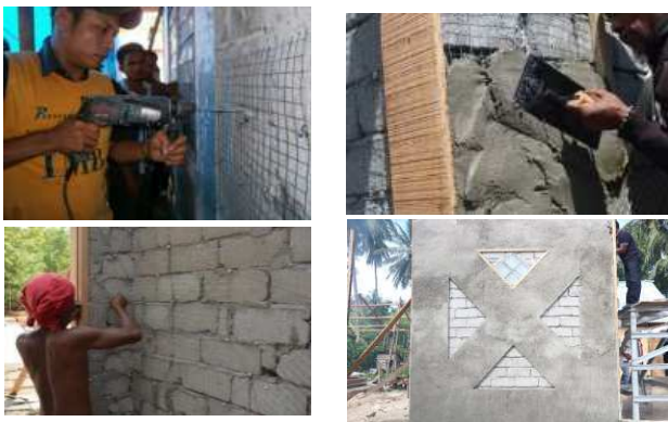
Fig. 3 Construction for Layer Ferrocement Reinforcement
