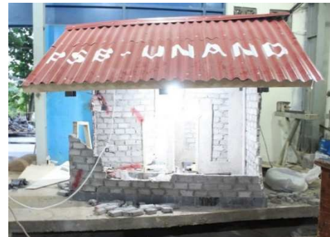
c. Condition of the Left Side of the Specimen
