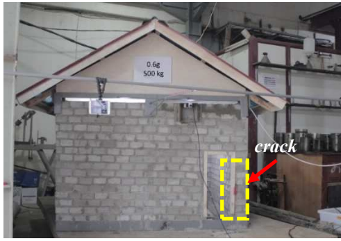
Fig. 14 The Condition of the Front of the Specimen at the time of an earthquake acceleration of 0.6 g
