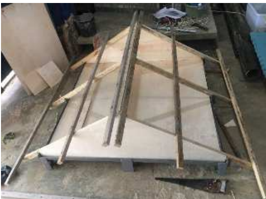
Fig. 10 Roof Truss Making Process
