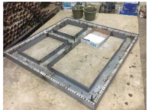
Fig. 6 Hollow Brick Wall Construction Process
