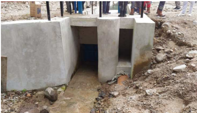
Fig. 3 Pipe Installation Inlet and Raw Water
