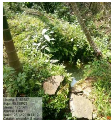
Fig. 3 Existing conditions of untreated septic tank discharge in Pantan Beunot subdistrict, Tiro Sub-district, Pidie district
